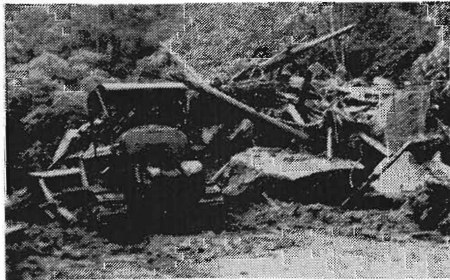
Flood damage on Range Road, Half way Creek 1958
